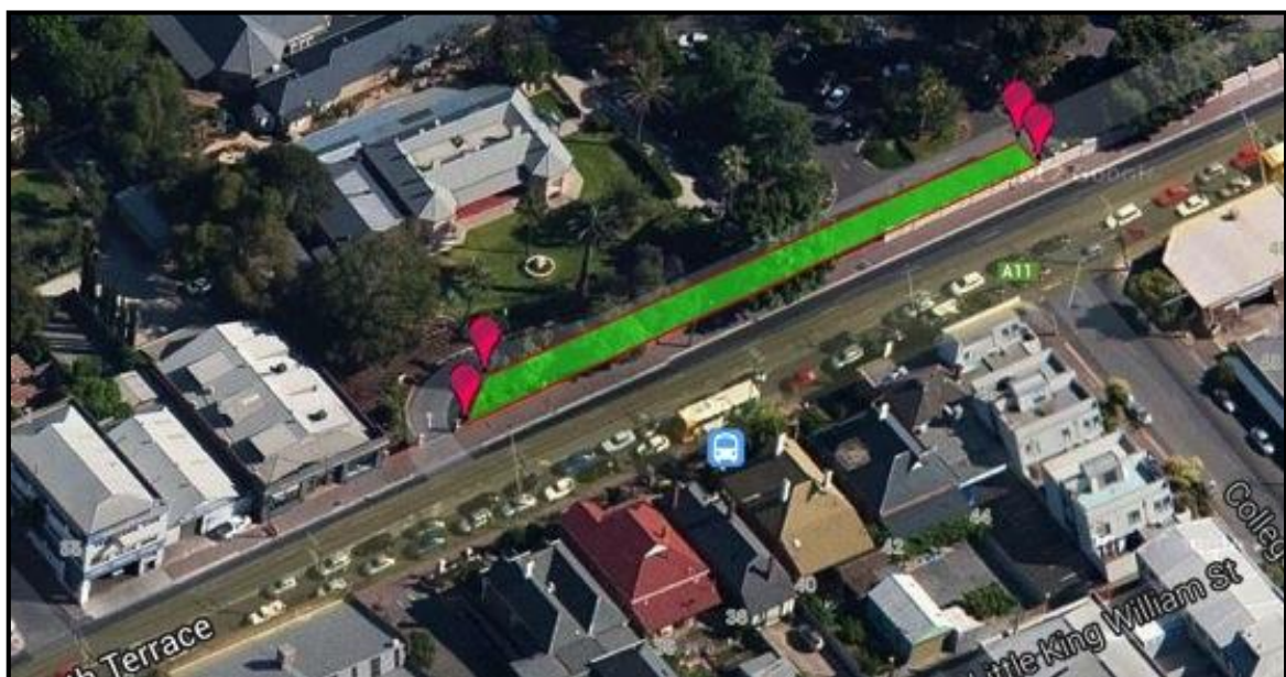
Figure 6: Area that could be used for bio-retention basin (in front of St Peter's College)
