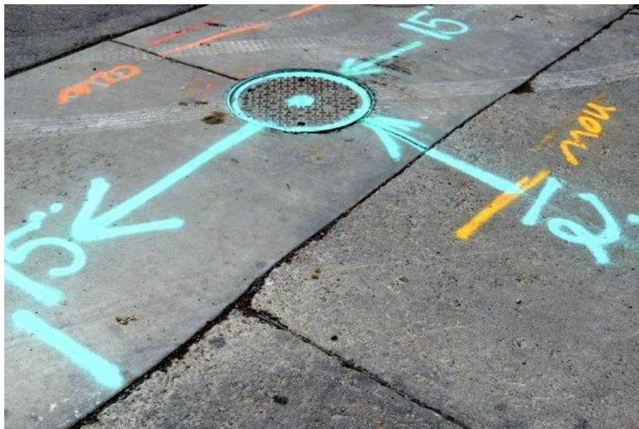
Figure 15 marking the location of underground service
