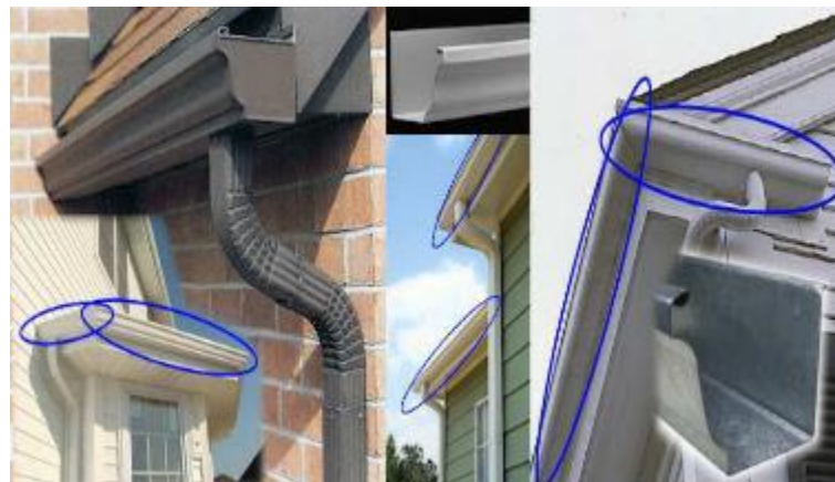
Figure 28: Examples of eaves gutter (hobbithouseinc 2015)
