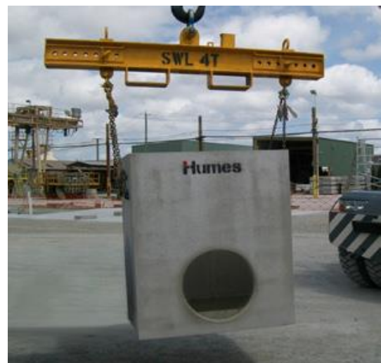
Figure 16 lifting a concrete pit (Humes 2012)
