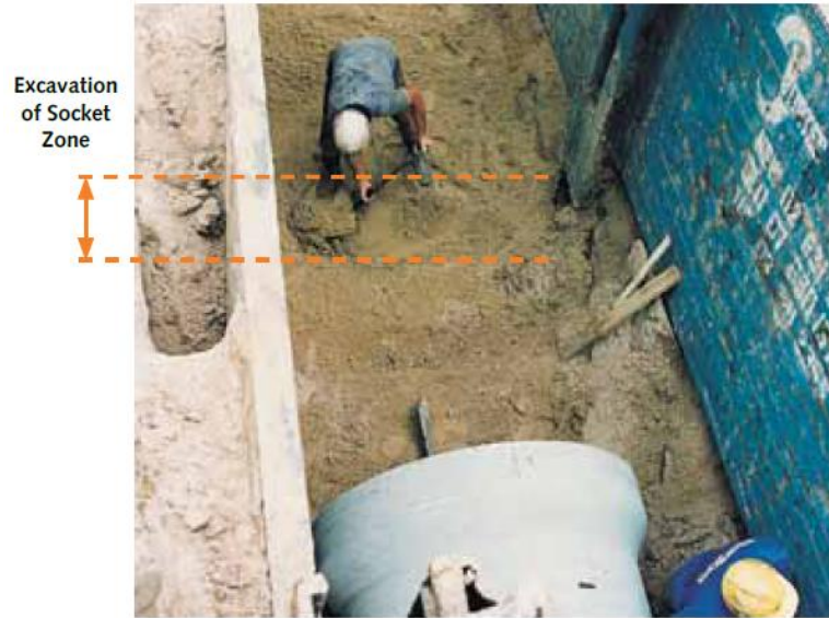
Figure 22: preparing the bedding for the pipe and pipe's socket (Humes, 2009)
