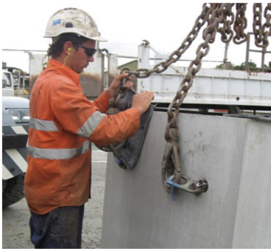
Figure 15 preparing a concrete pit prior to lifting
