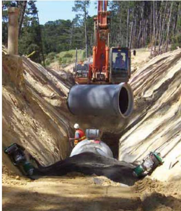
Figure 21 lowering a concrete pipe into a trench (Humes 2009)
