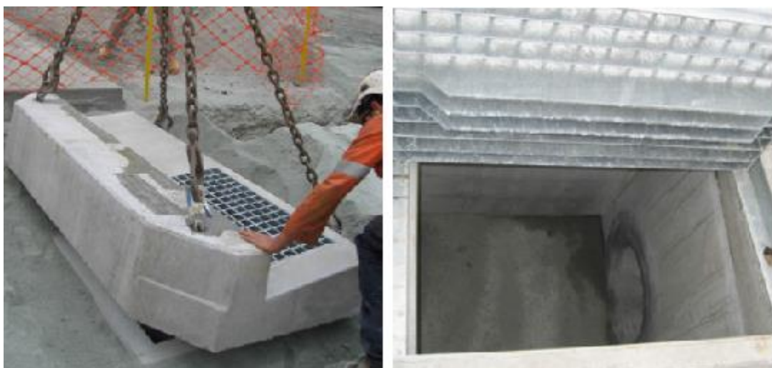
Figure 20: Side Entry Pit Installation (Humes 2012)
