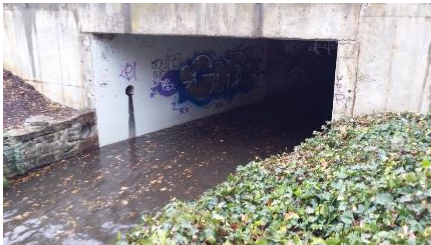
Figure 82: Concrete Box Culvert beneath Hackney Road, the start of Section 5 (Hydro-future 2015)
