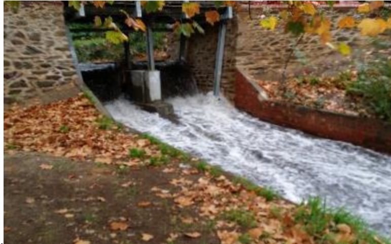
Figure 75: Photo of the Weir, which is used to decrease the velocity of the water to assist in erosion control (Hydro-Future 2015)
