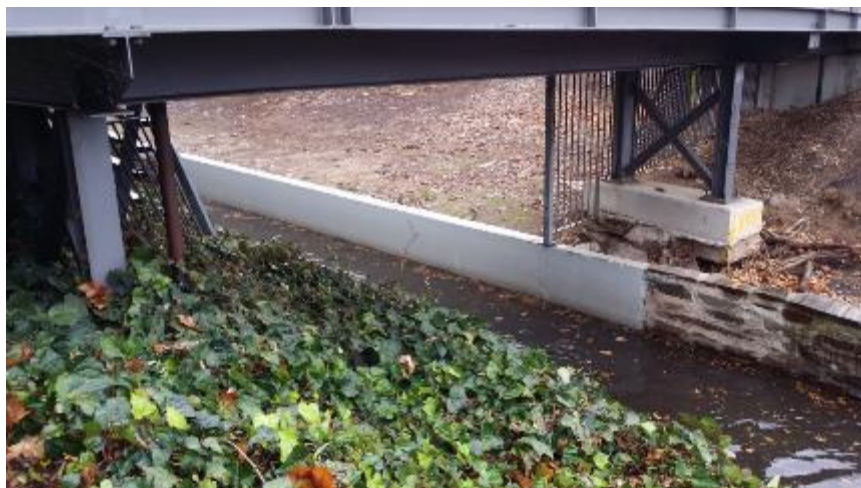
Figure 83: Typical Creek Profile in Section 5 (Hydro-Future 2015)
