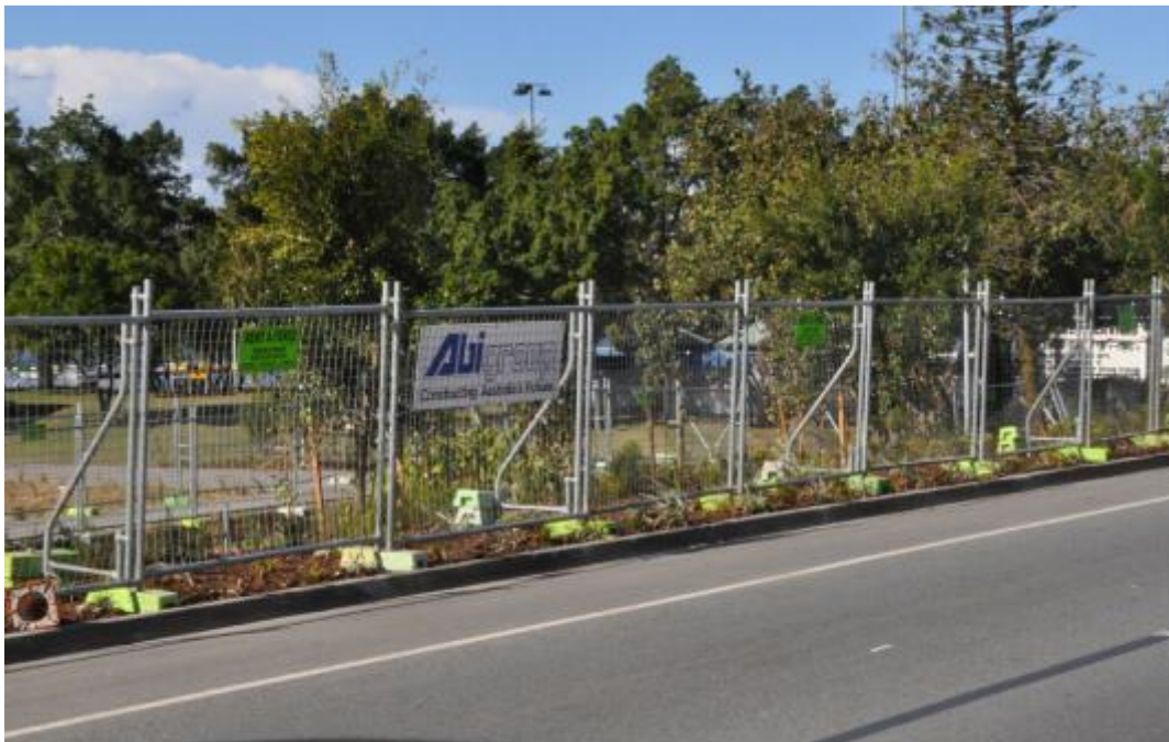
Figure 236 Temporary Mesh Fencing
