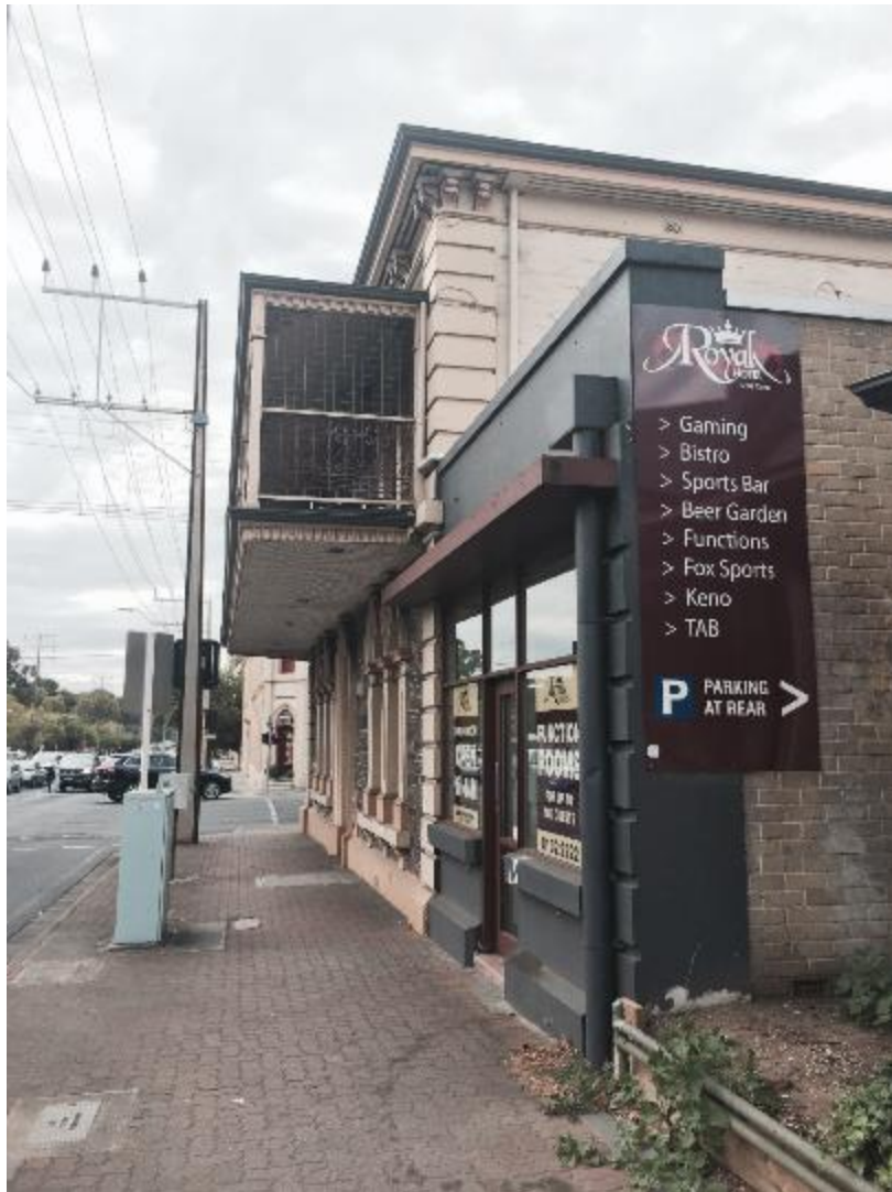
Figure 211 2 North Terrace Kent Town, SA (Hydro-Future, 2015)
