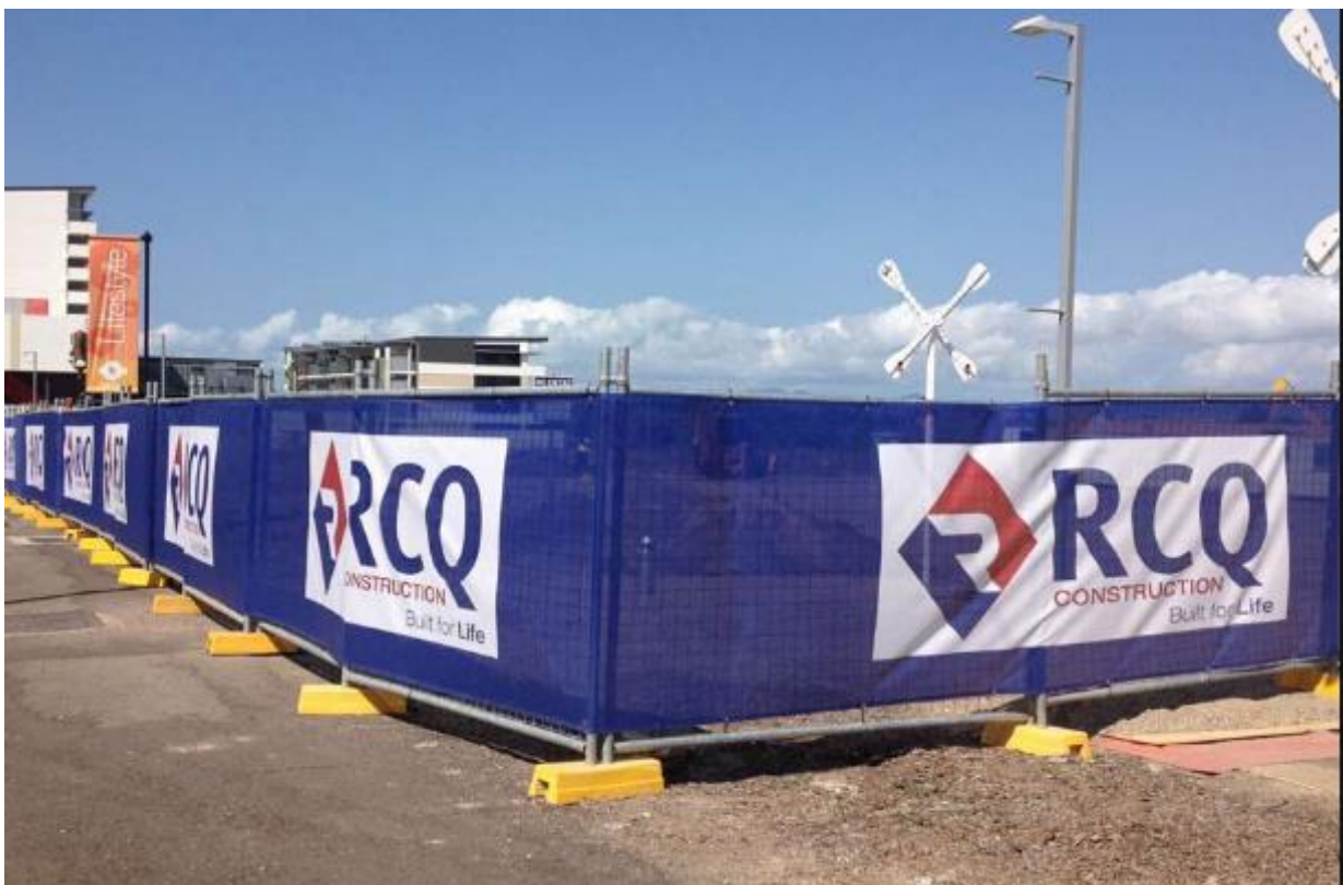
Figure 237 temporary mesh fencing with cloth cover
