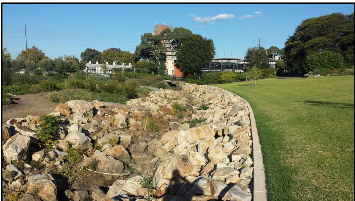
Figure 11 - Photo of First Creek showing wider channel and rock-lined bed
