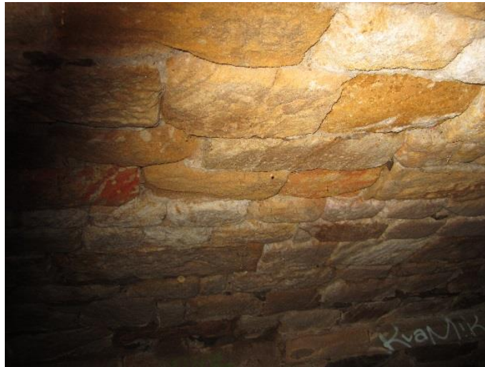
Figure 44: Visual inspect of mortar integrity (Hydro-Future, 2015)
