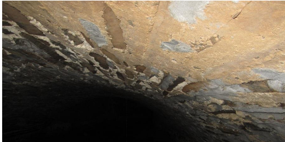
Figure 45 – Sandstone Culvert mortar repair (Hydro-Future, 2015)
