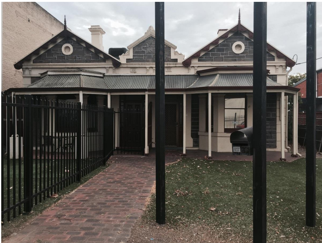
Figure 33: 33 North Terrace HACKNEY, SA - Heritage Building (Hydro-Future, 2015)
