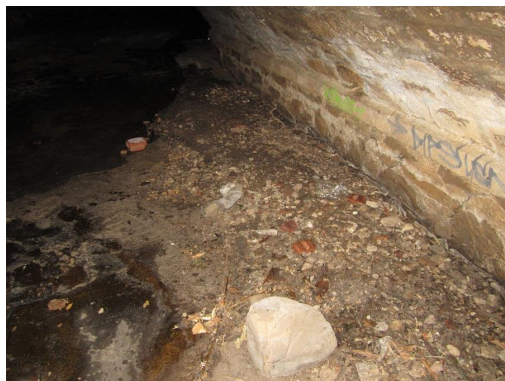
Figure 42: Visual inspect of culvert condition (Hydro-Future, 2015)
