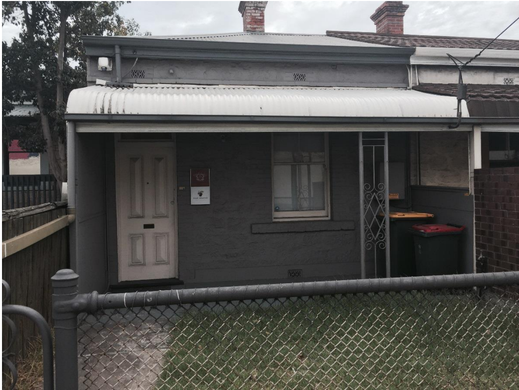
Figure 32: 37 North Terrace Hackney, SA - Heritage Building (Hydro-Future, 2015)
