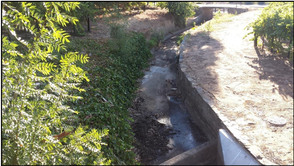
Figure 9 – First Creek, note the Concrete and Stone Retaining Wall (Hydro-Future, 2015)
