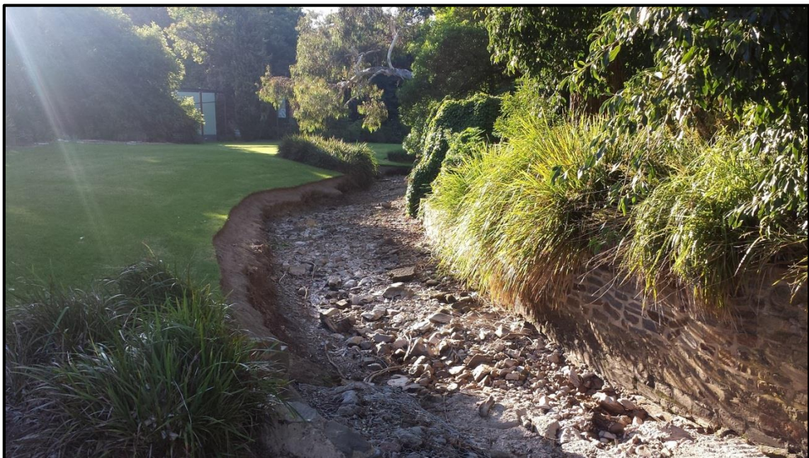
Figure 13: Photo of First Creek Showing Erosion
