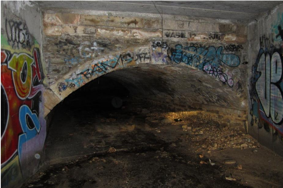
Figure 40 - Sandstone Culvert – Box Culvert Connection (Hydro-Future, 2015)
