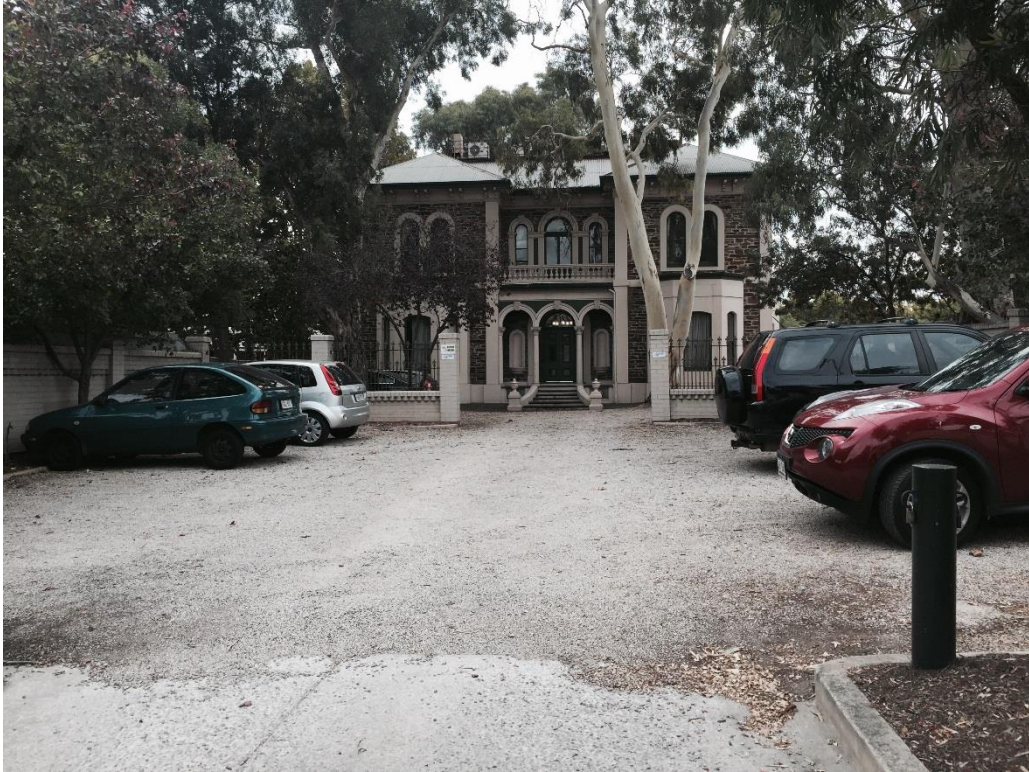
Figure 34: 23 North Terrace Hackney, SA - Heritage Building (Hydro-Future, 2015)
