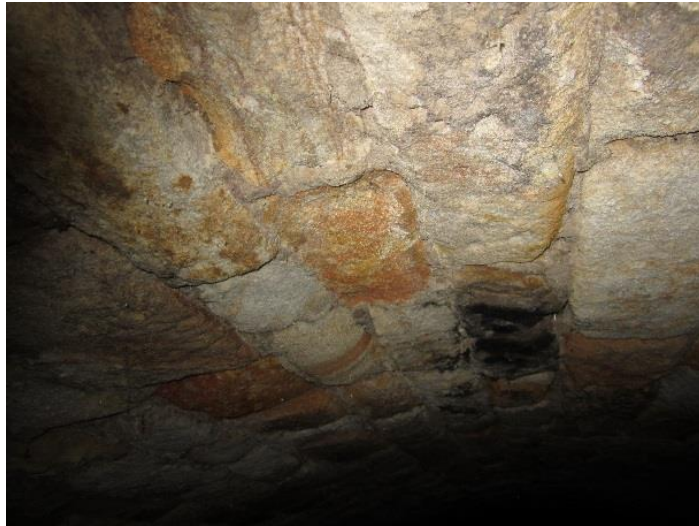
Figure 43: Visual inspect of mortar integrity (Hydro-Future, 2015)
