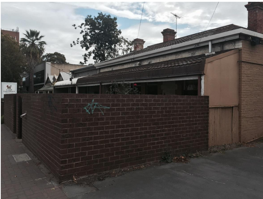
Figure 35: 39 and 41 North Terrace Hackney, SA - Heritage Building (Hydro-Future, 2015)
