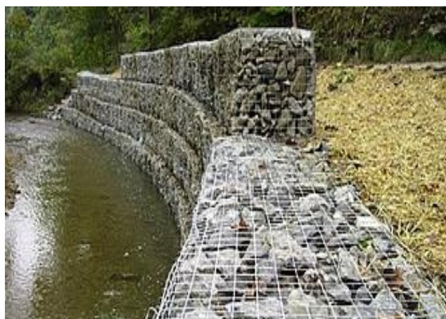
Figure 128: Gabion Wall (Sahero Gabion Barrier n.d.).
