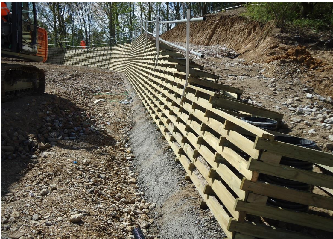
Figure 127: Crib Wall (Phi Group 2015)
