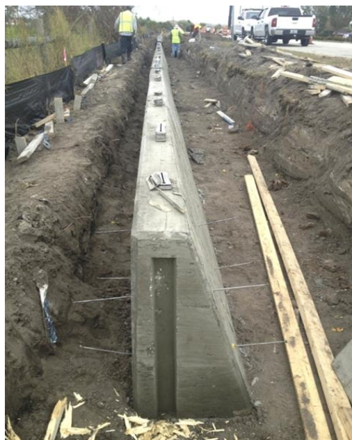
Figure 125: Gravity Retaining Wall (ROADWAY, n.d.)
