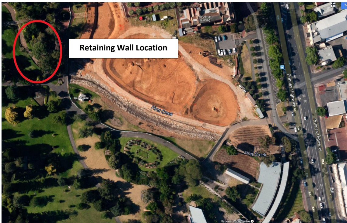
Figure 119: retaining Wall Location (Hydro-Future, 2015)
