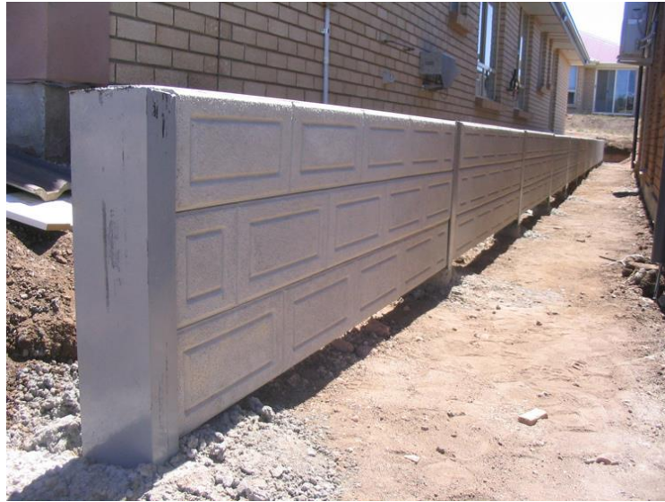
Figure 123: Concrete Retaining Wall (Brislandscaping, 2015)
