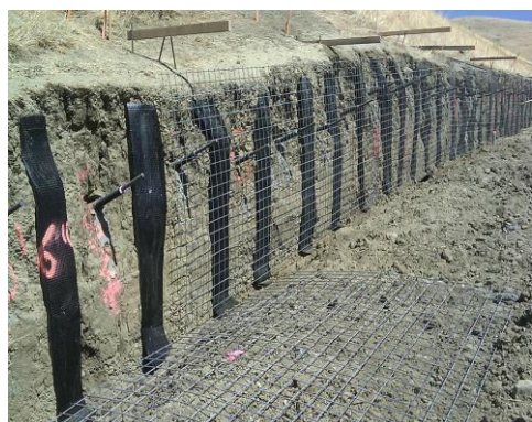
Figure 130: Soil Nail Wall (Kutschke, Tarquinio & Petersen 2007)
